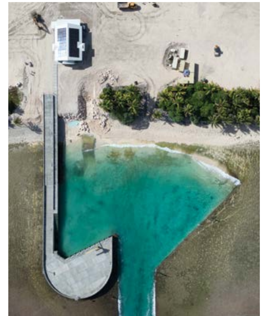
Image: The new climate-resilient harbour on Niutao island, co-funded by the AIFFP and ADB.
