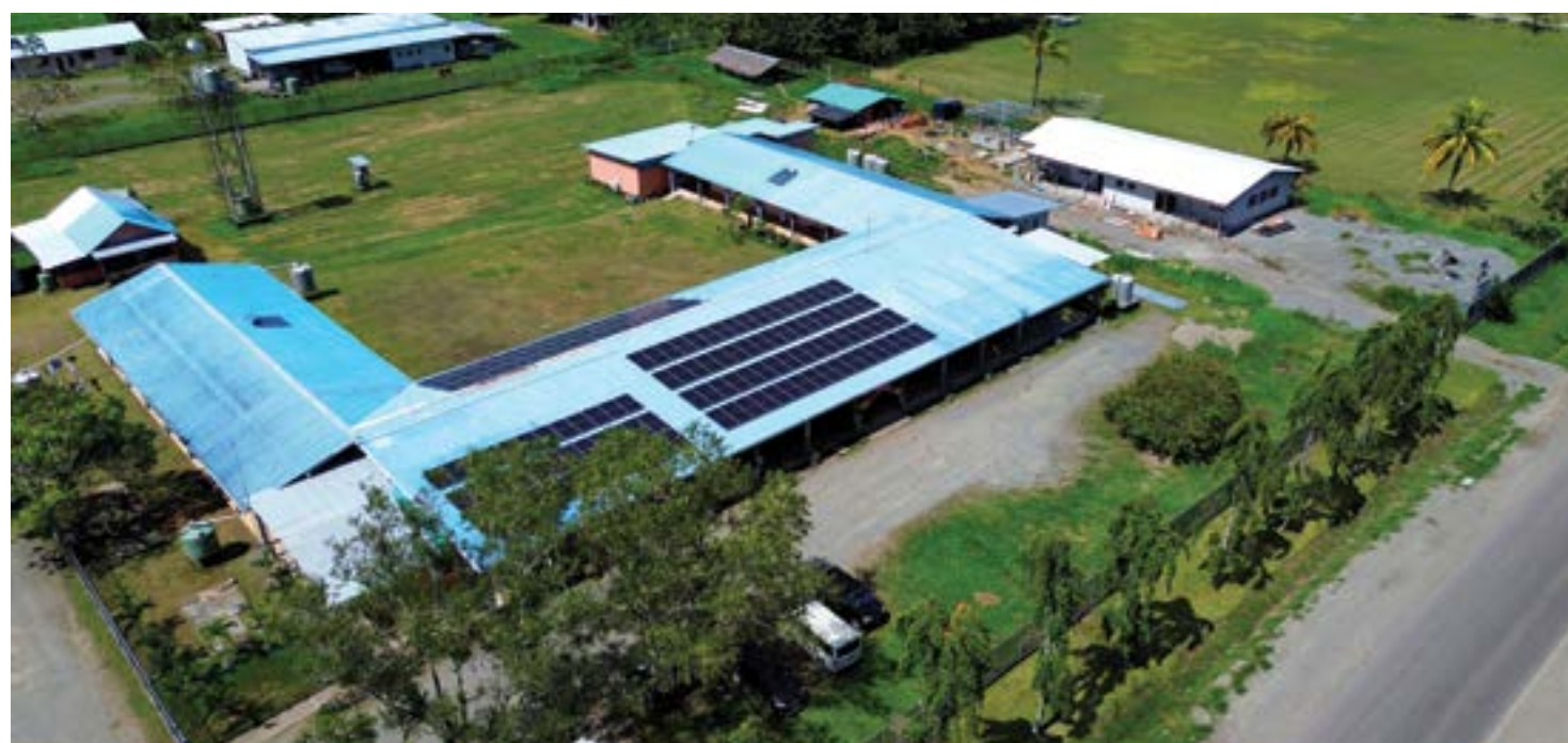
Image: The hybrid solar-battery-diesel system is producing reliable and free power for Good Samaritan Hospital in Guadalcanal Province, Solomon Islands.
