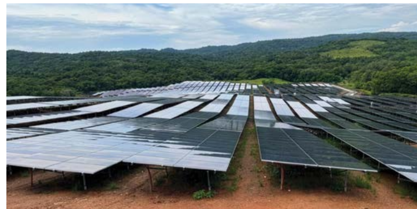
Image: Palau's first utility-scale solar power plant at Ngatpang on Babeldaob opened in June 2023.
