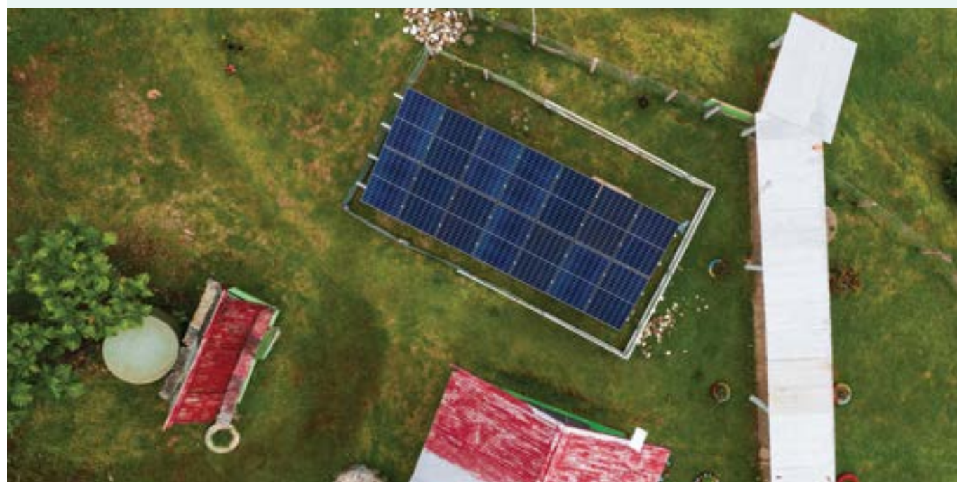
Image: Rabi Island's Buakonikai Primary School now has a reliable, solar-powered energy system.
